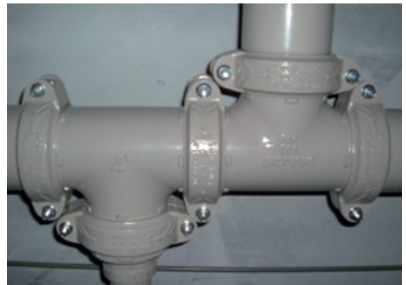
Evergreen Aviation Hangar 2, Tainan, Taiwan
