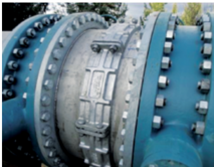
Model R-88 Couplings with stainless steel rings used on stainless steel hydro electric pipe line, BC, Canada.
