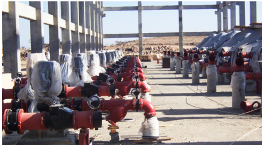
HVAC plant room, King Khaled University, Abha, Kingdom of Saudi Arabia
